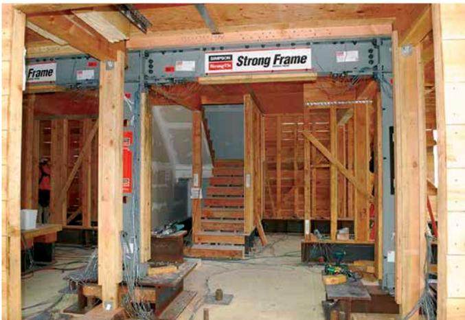
Part of a steel special moment frame installed as a retrofit in the soft-story test building at UCSD.
